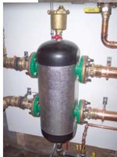
*Off-the-shelf low-loss-header solutions can be accomplished two ways: (1) for light-commercial applications up to about 250 MBH, with closely spaced tees (above) and, (2) for larger systems, with a hydraulic separator (left).*
